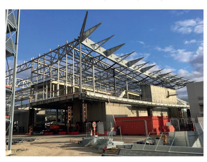
technical walkways hanging from the roof. This structure carries the loads of the sub-structure of the facade cladding in perforated sheet made with spatial lattices.
